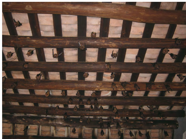
Figure 42. A roost of H. armiger in an abandoned building.
